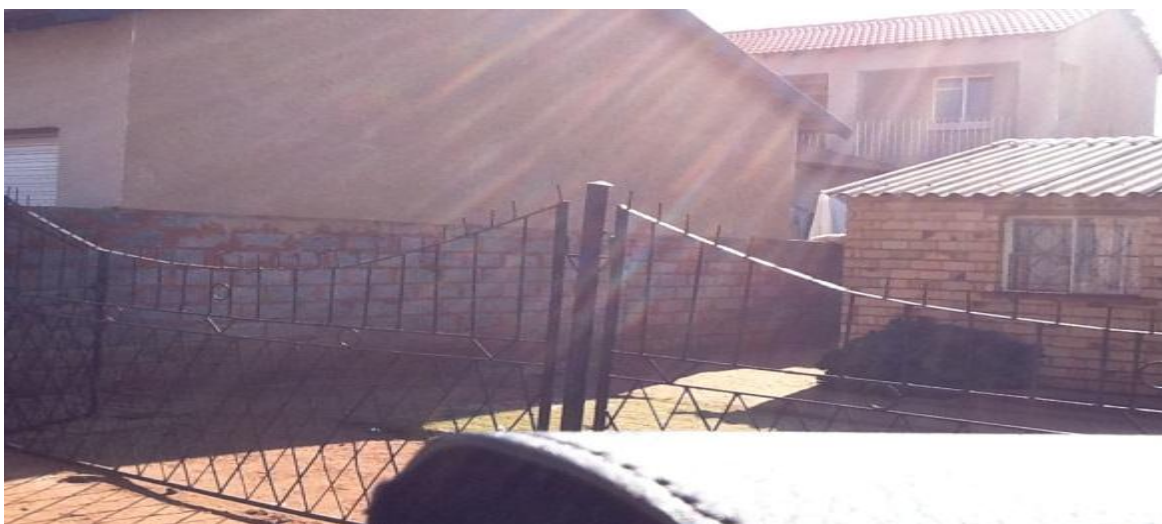
Figure 6: The Mfuku house (on the left) has been transformed from a house that looked like the one on the right to a double-storey structure comprising 4 bedrooms, 2 bathrooms and 2 toilets
